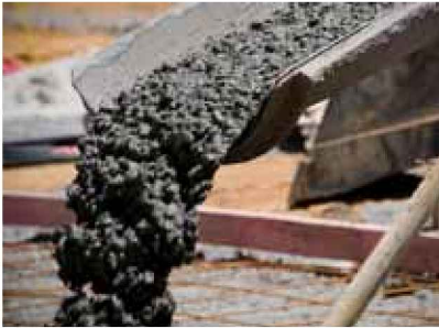
Pouring reinforced concrete
