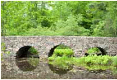
A masonry footbridge
